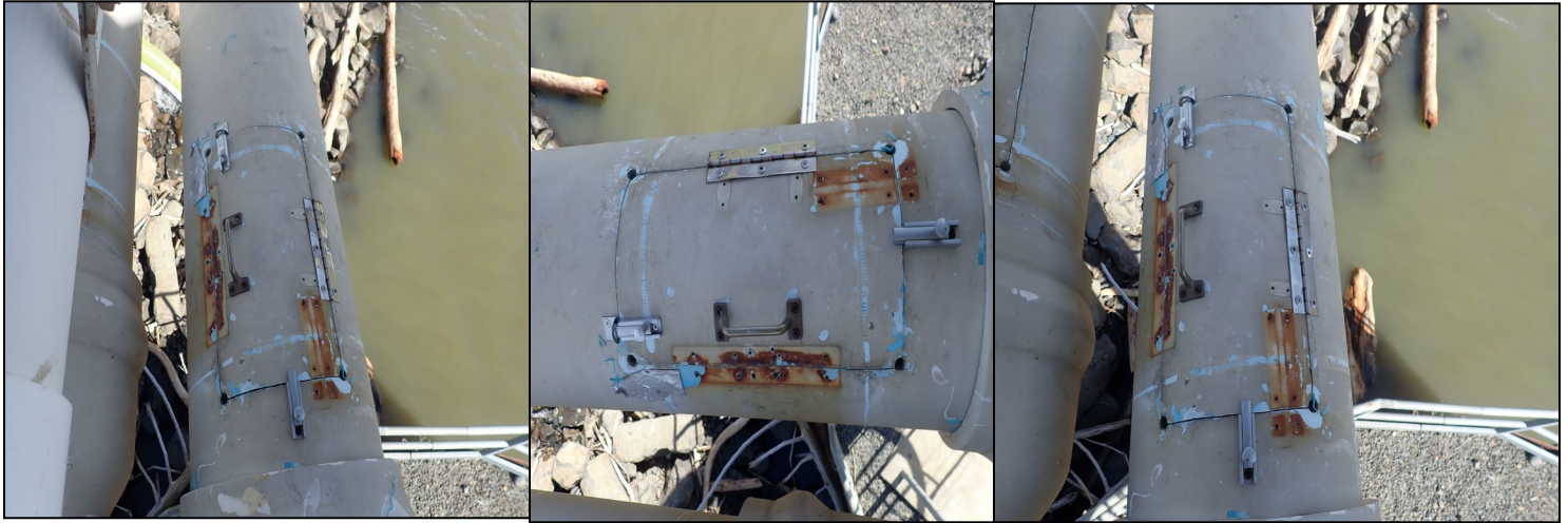
Cleanout hatch condition after hardware installation
